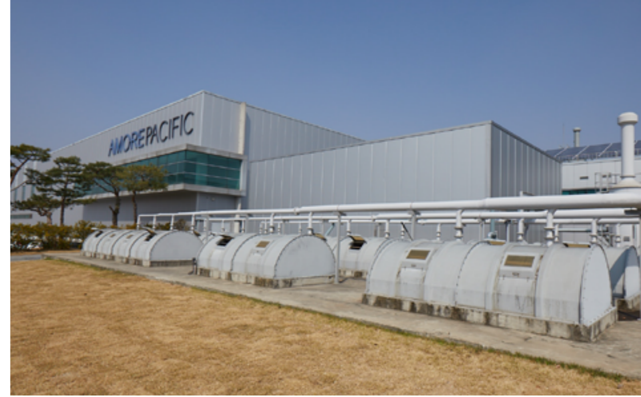
Rainwater repository at Osan Amore Beauty Park
